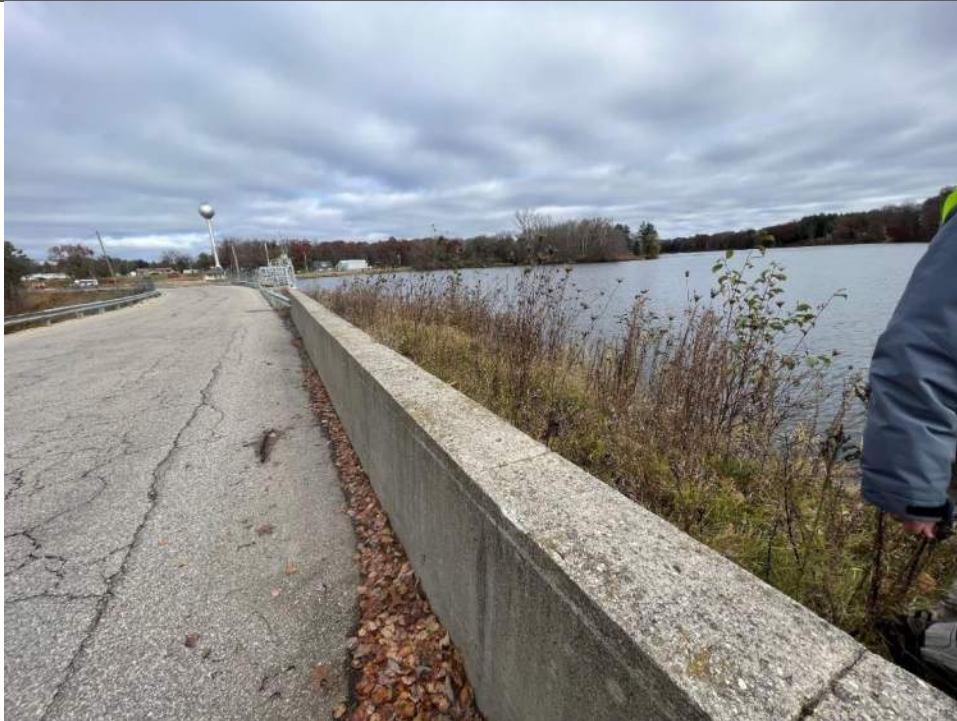
Photo No. 78 – Upstream Left Embankment Flood Wall - Looking Right
