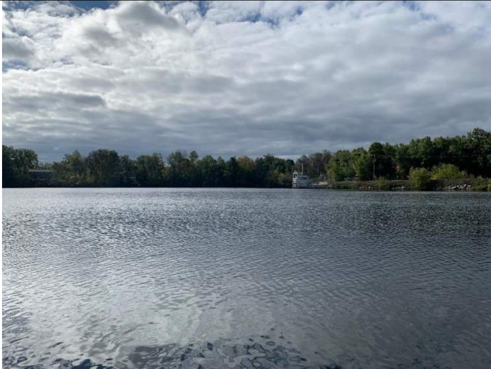
Photo No. 63 – Primary Spillway – Impoundment Looking Downstream
