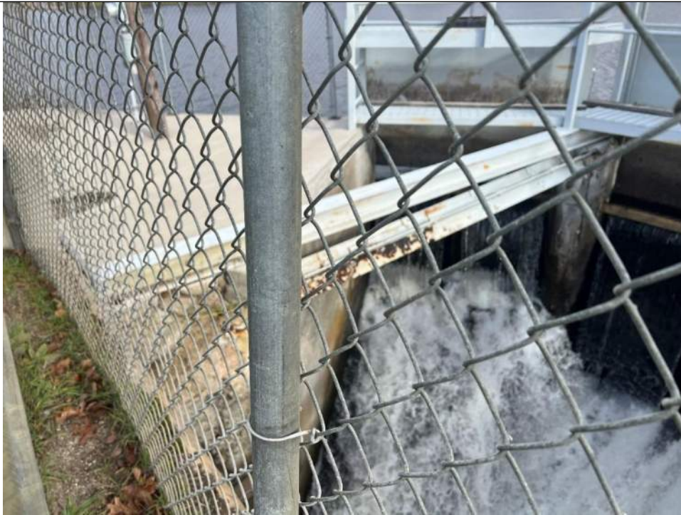
Photo No. 61 – Right Gate of Primary Spillway – Looking Upstream
