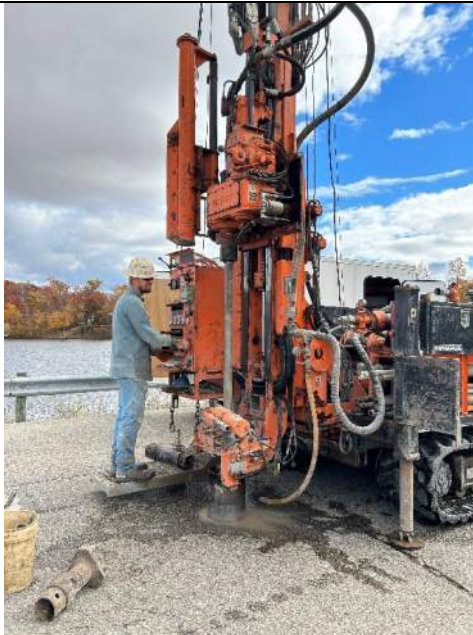
Photo No. 1 – Pearson Drilling Starting Boring B-01 by Coring through HMA and RCC
