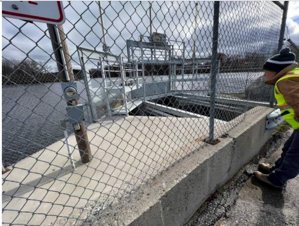
Photo No. 56 – Primary Spillway – Looking Upstream
