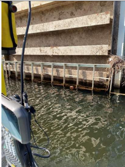
Photo No. 68 – Left Primary Spillway – Impoundment Looking Downstream
