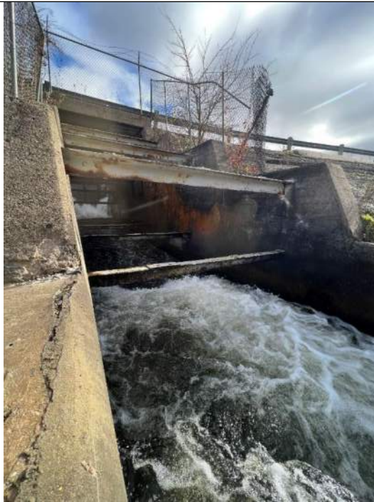
Photo No. 45 – Outlet of Primary Spillway – Looking Upstream
