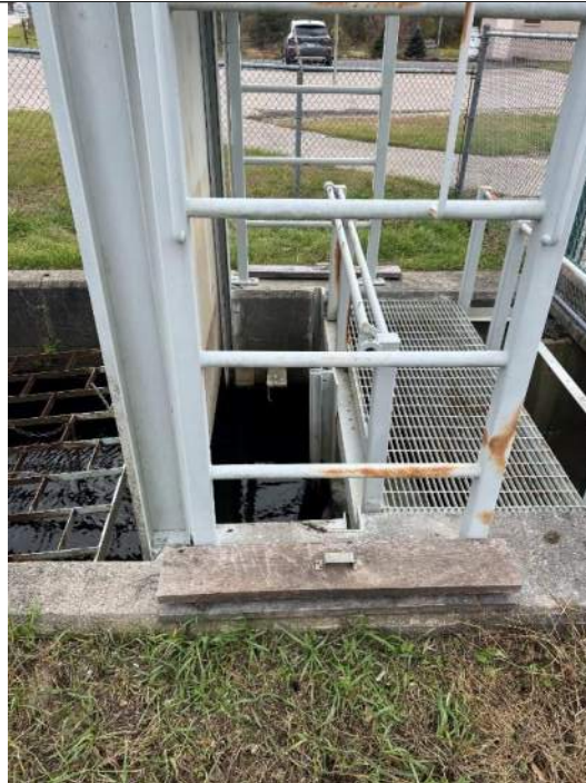
Photo No. 4 – Auxillary Spillway – Gate and Operator Deck
