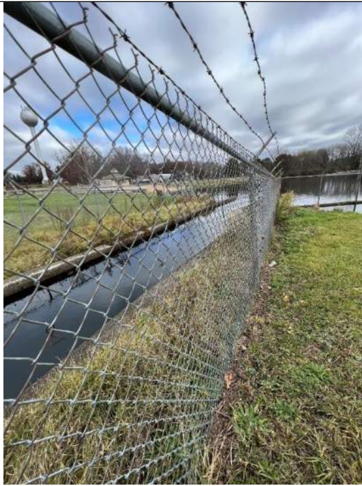
Photo No. 13 – Auxillary Spillway – Upstream of Road Looking Upstream
