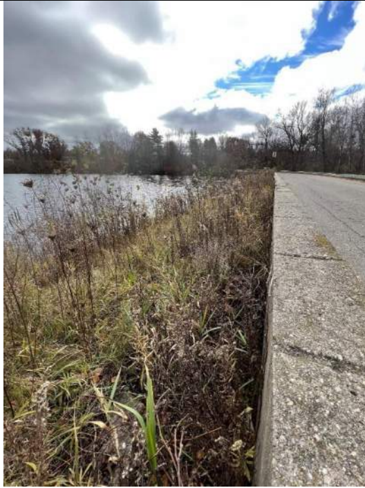
Photo No. 75 – Upstream Left Embankment Flood Wall - Looking Left
