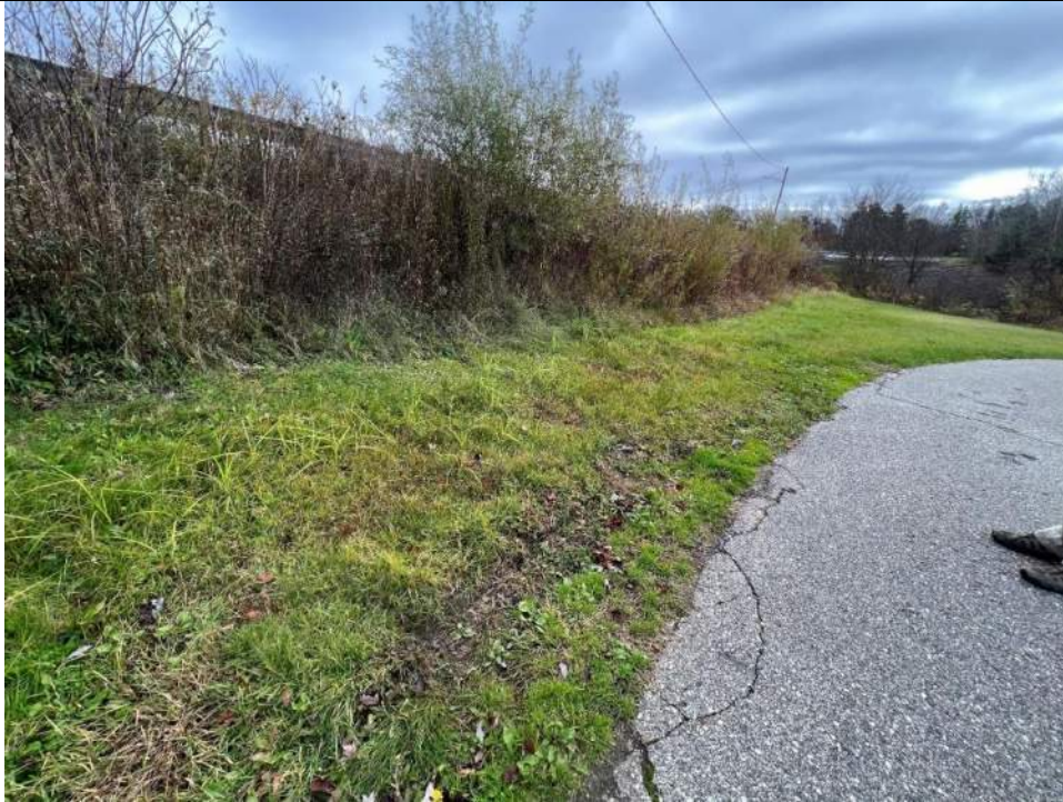
Photo No. 25 – Right Embankment – Downstream Toe Looking Upstream
