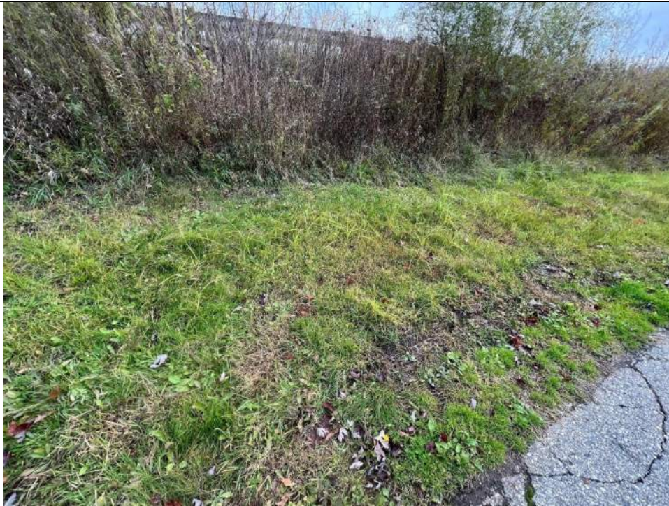
Photo No. 23 – Right Embankment – Downstream Toe Looking Upstream
