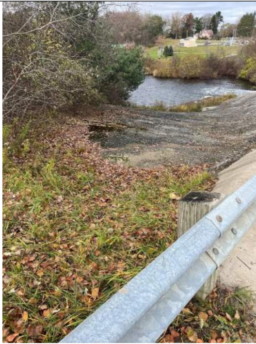
Photo No. 83 – Downstream Left Embankment RCC Slope
