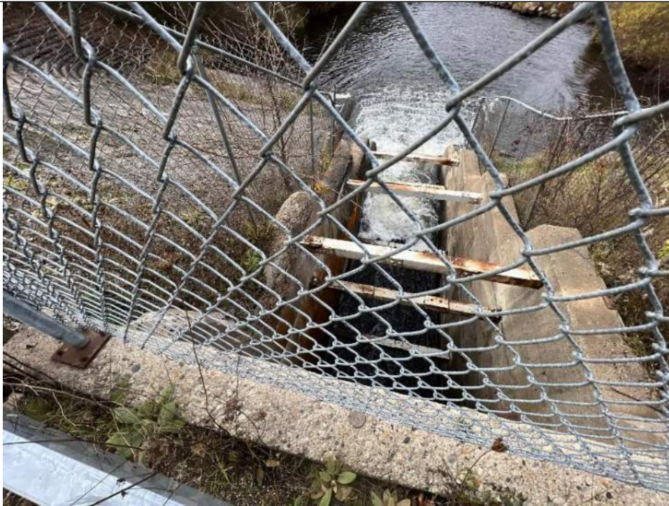
Photo No. 93 – Primary Spillway Outlet – Looking Downstream
