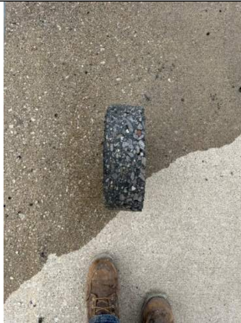
Photo No. 3 – Side/Section of RCC Core from B-01
