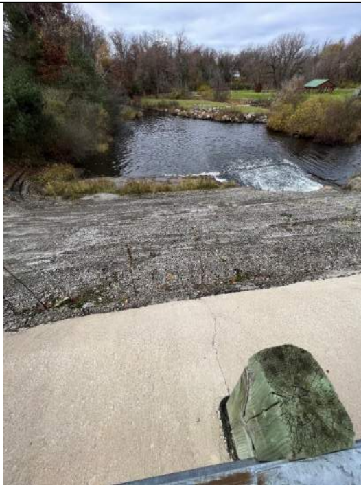
Photo No. 88 – Downstream Left Embankment RCC Slope – Looking Downstream
