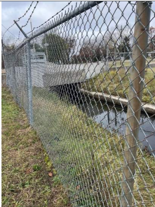
Photo No. 14 – Auxillary Spillway – Upstream of Road Looking Downstream
