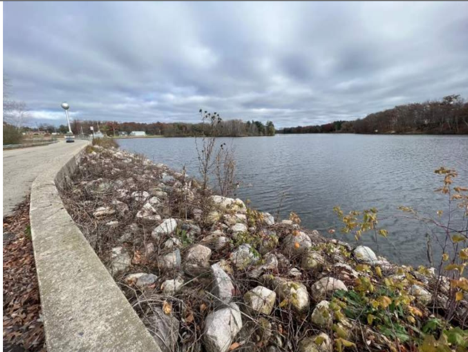
Photo No. 82 – Upstream Left Embankment Flood Wall - Looking Right
