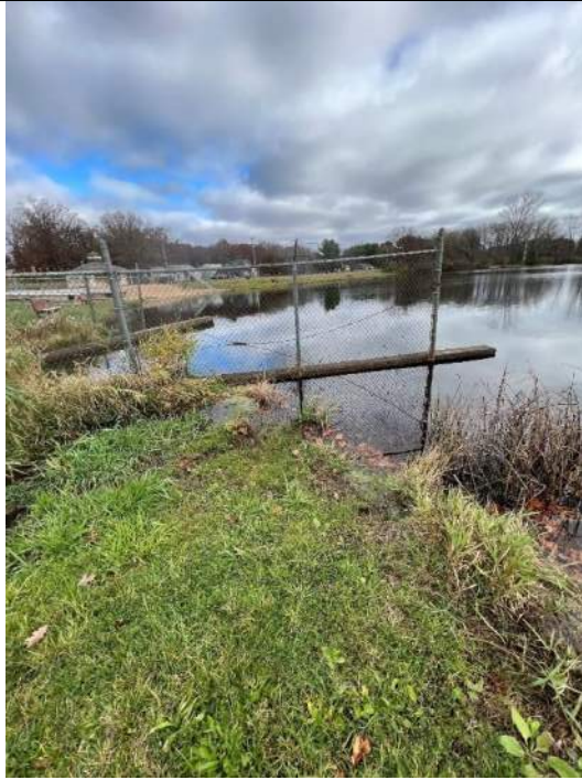
Photo No. 11 – Auxillary Spillway – Upstream of Road Looking Upstream
