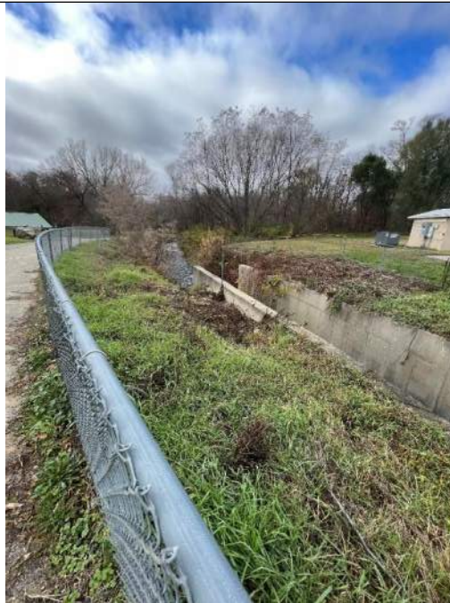
Photo No. 3 – Auxillary Spillway – Downstream of Road Looking Downstream
