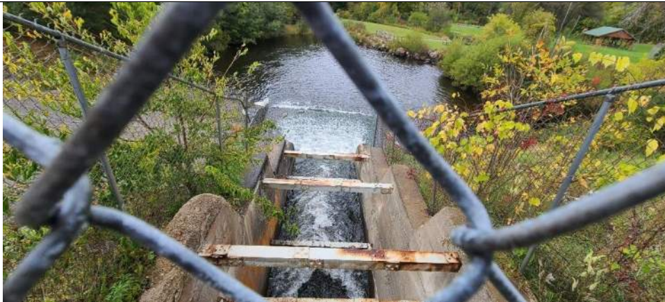
Photo No. 94 – Primary Spillway Outlet – Looking Downstream
