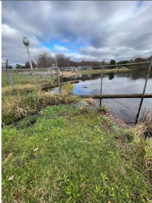
Photo No. 10 – Auxillary Spillway – Upstream of Road Looking Upstream
