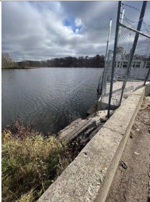
Photo No. 50 – Right Upstream Flood Wall at Primary Spillway Right Abutment
