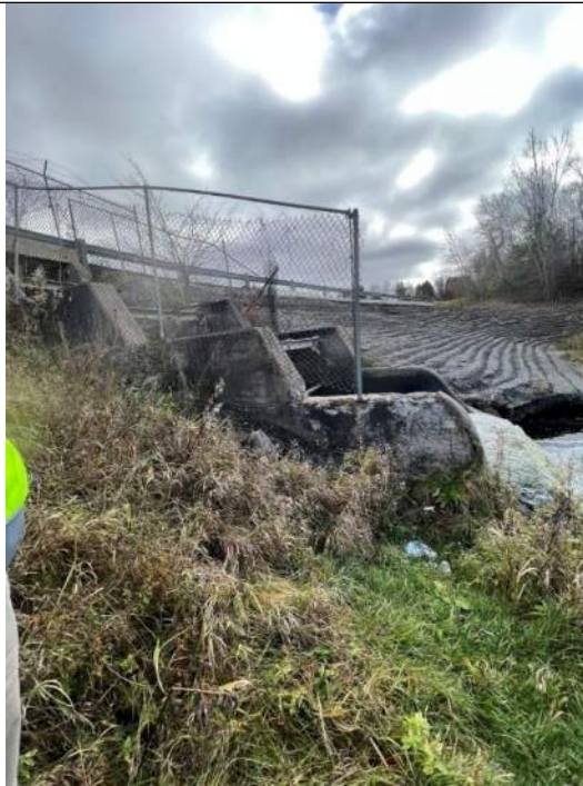
Photo No. 41 – Right Downstream Primary Spillway Wall
