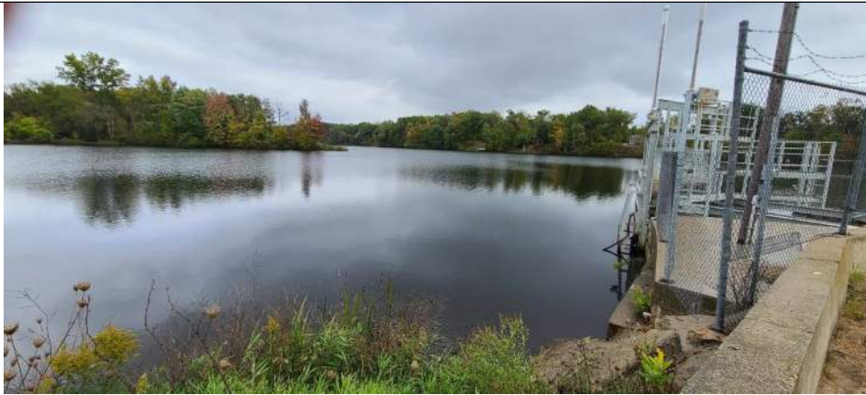
Photo No. 51 – Right Primary Spillway Abutment Looking Upstream
