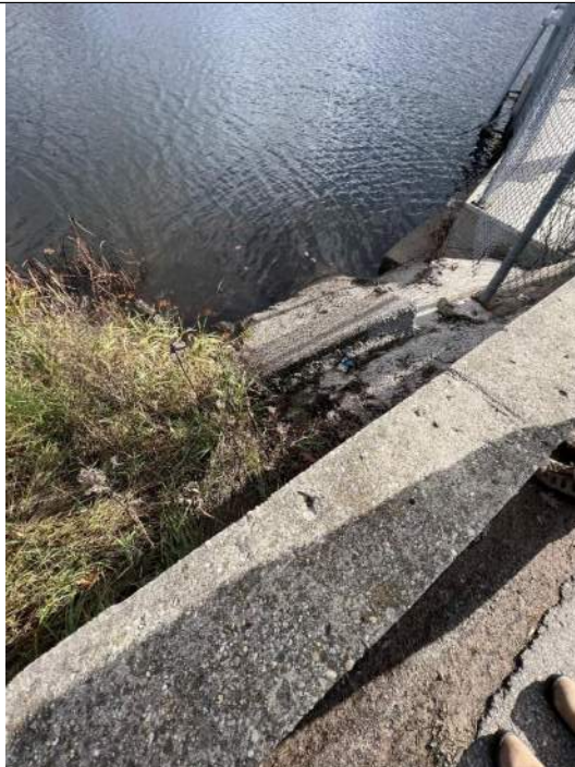
Photo No. 52 – Right Primary Spillway Abutment
