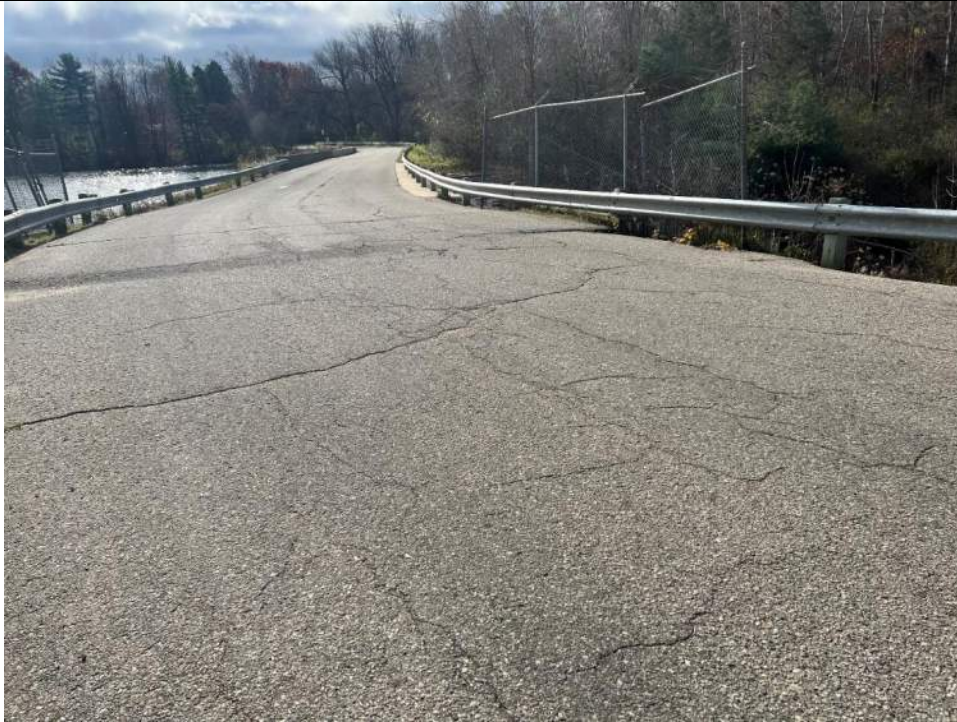
Photo No. 53 – Roadway over Primary Spillway – Looking Left
