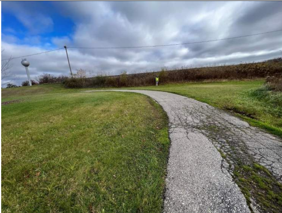
Photo No. 29 – Right Embankment – Downstream Toe Looking Upstream
