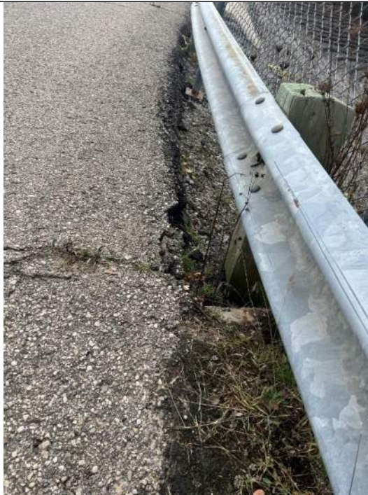
Photo No. 95 – Guardrail Post Embedment at Primary Spillway Downstream Side of Crest – Looking Downstream
