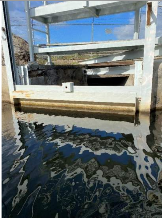
Photo No. 69 – Left Primary Spillway – Impoundment Looking Downstream
