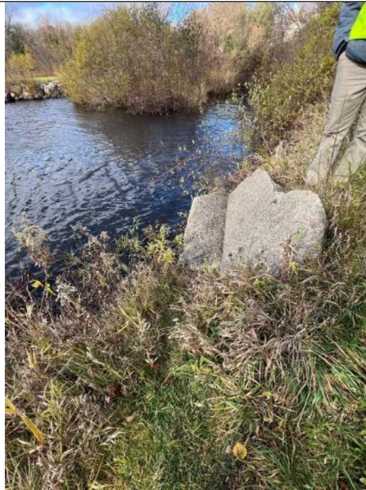
Photo No. 47 – Downstream Toe of Right Embankment – Looking Downstream
