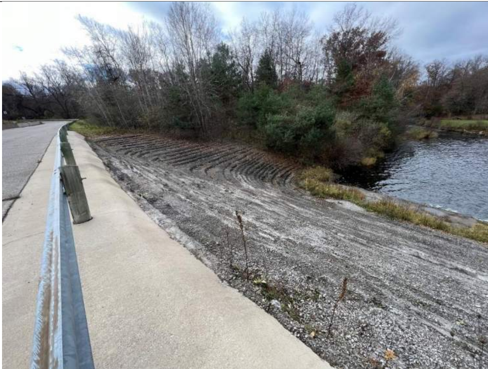
Photo No. 90 – Downstream Left Embankment RCC Slope – Looking Left
