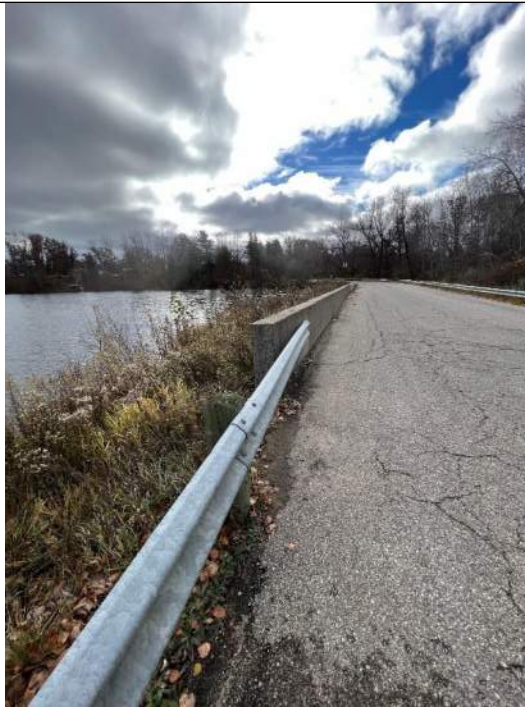
Photo No. 73 – Interface of Upstream Side of Left Embankment at Overtopping Section and Flood Wall – Looking Left
