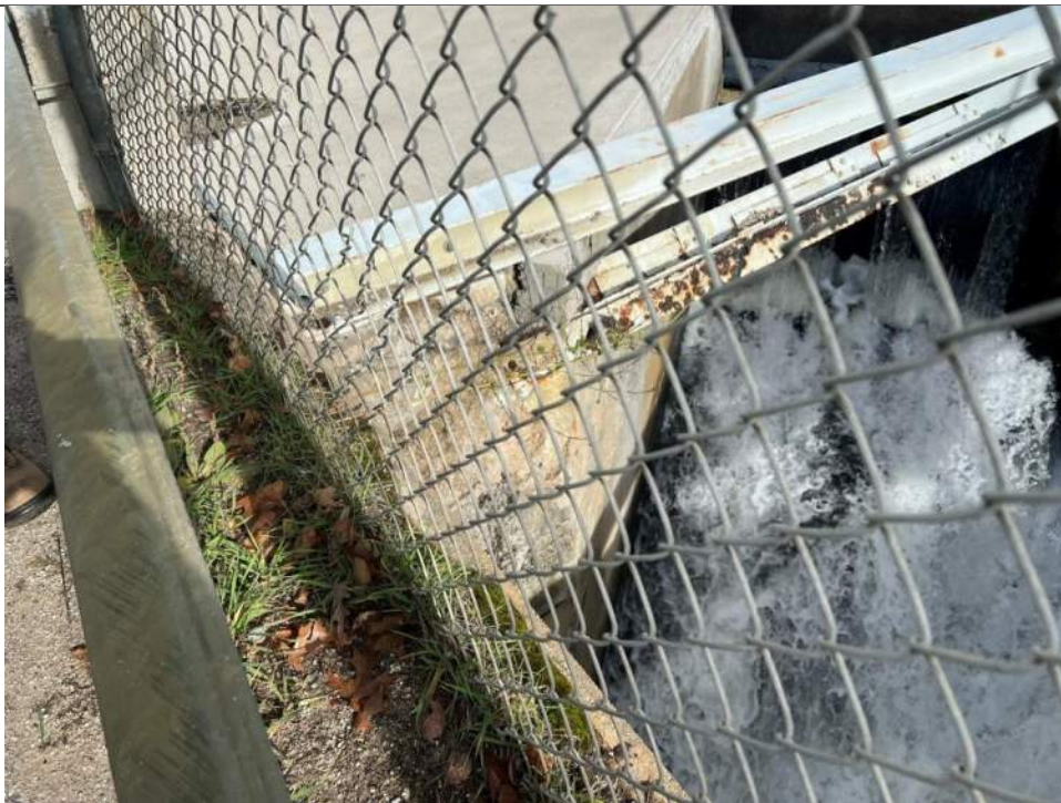
Photo No. 58 – Downstream End of Right Primary Spillway Brace – Looking Right
