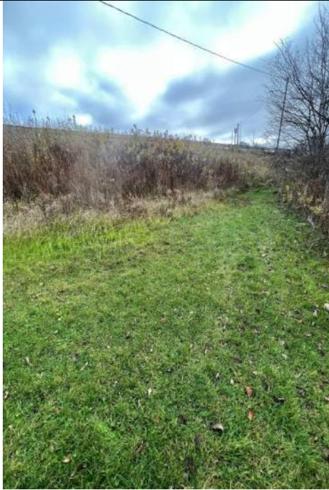
Photo No. 33 – Right Embankment – Downstream Toe Looking Left
