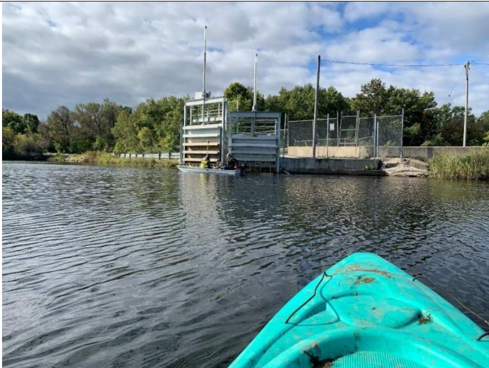
Photo No. 64 – Right-Side of Primary Spillway – Impoundment Looking Downstream
