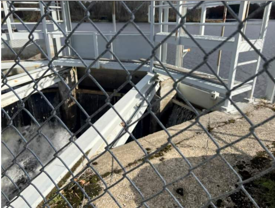
Photo No. 59 – Left Primary Spillway Brace – Looking Upstream
