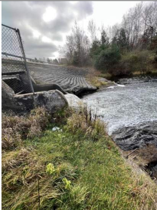
Photo No. 37 – Outlet of Primary Spillway
