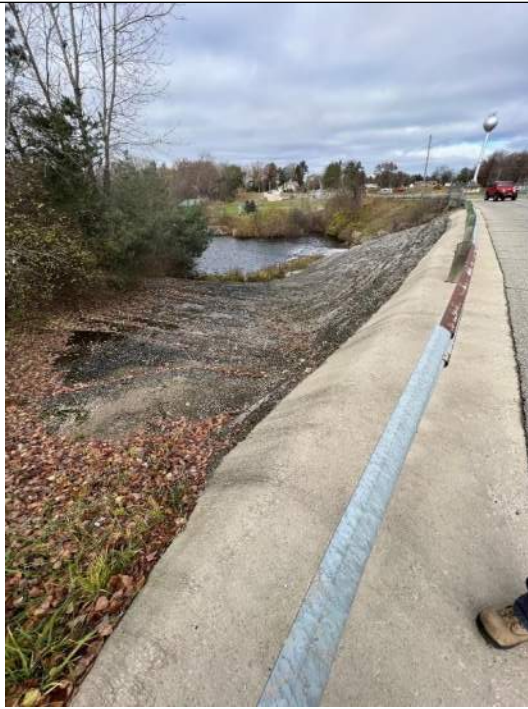
Photo No. 85 – Downstream Left Embankment RCC Slope – Looking Downstream
