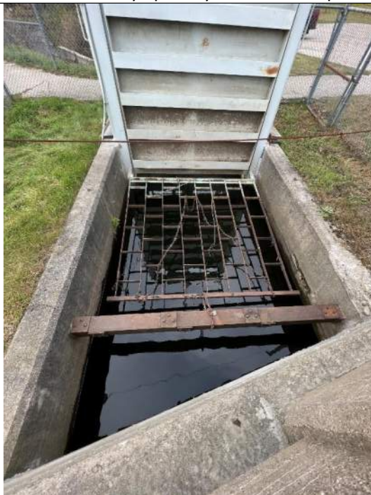
Photo No. 6 – Auxillary Spillway – Trashrack Looking Downstream
