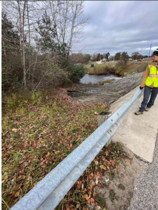
Photo No. 84 – Downstream Left Embankment RCC Slope – Looking Downstream
