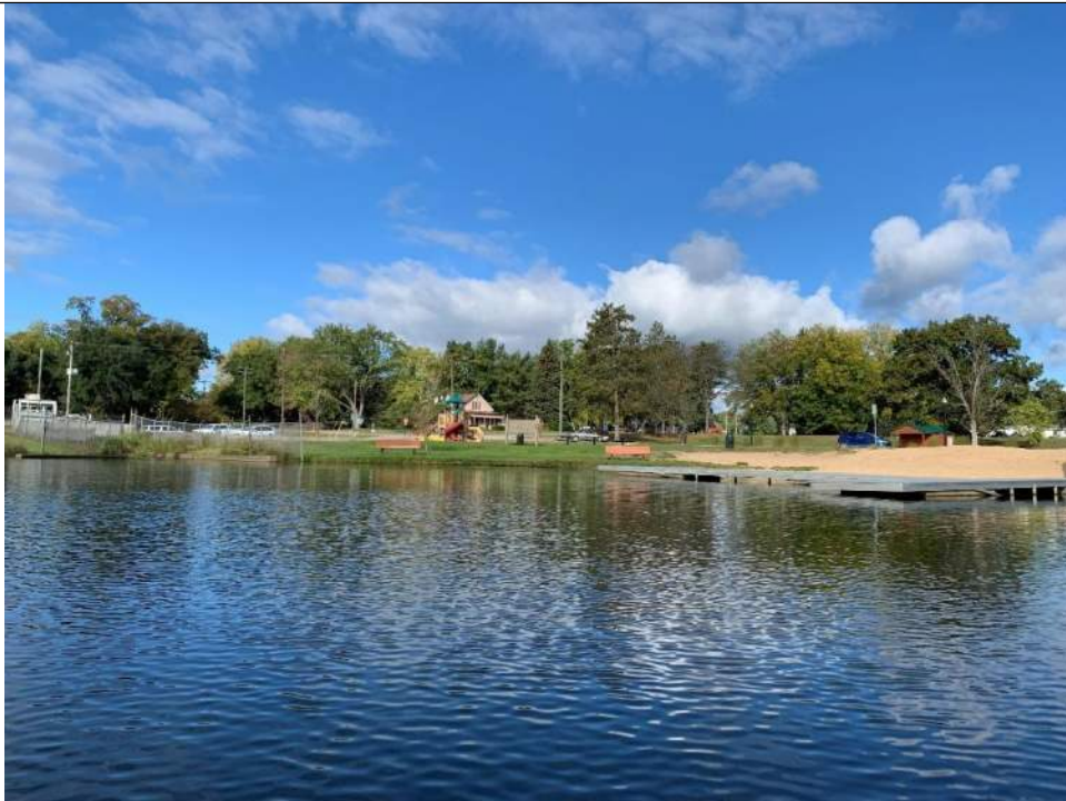
Photo No. 18 – Auxiliary Spillway, Playground and Beach – Impoundment Looking Downstream
