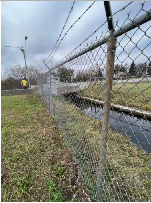
Photo No. 15 – Auxillary Spillway – Upstream of Road Looking Downstream
