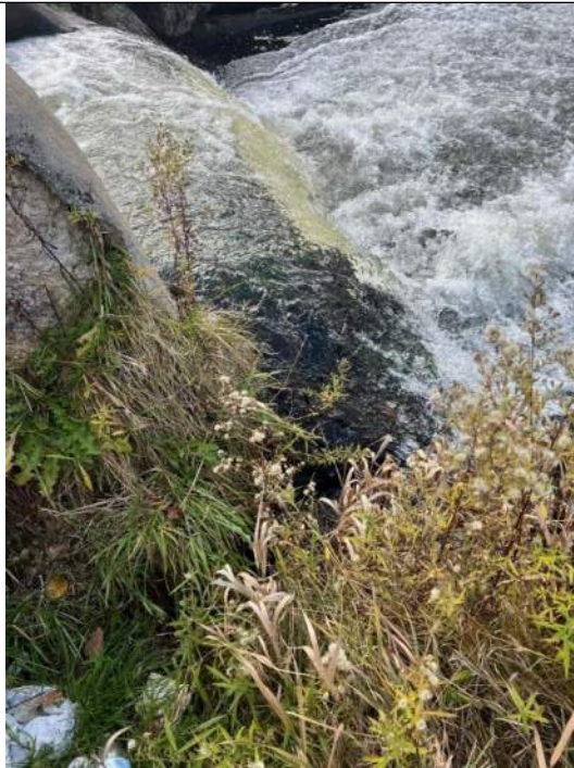
Photo No. 43 – Outlet of Primary Spillway
