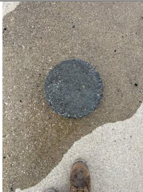
Photo No. 2 – Top of RCC Core from B-01
