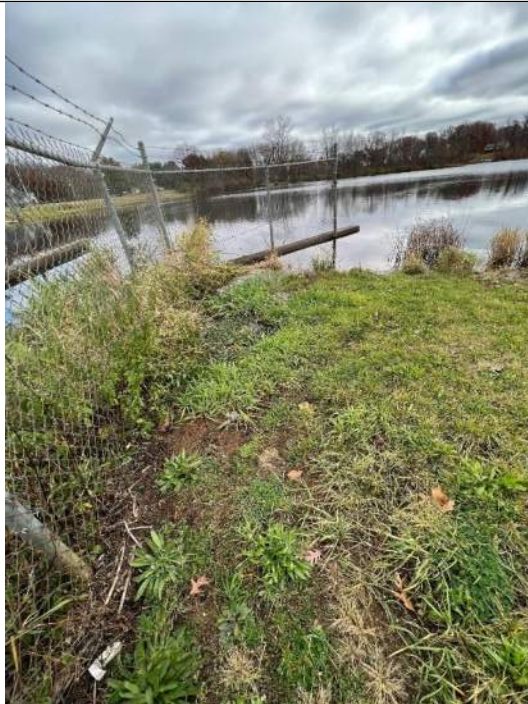
Photo No. 12 – Auxillary Spillway – Upstream of Road Looking Upstream
