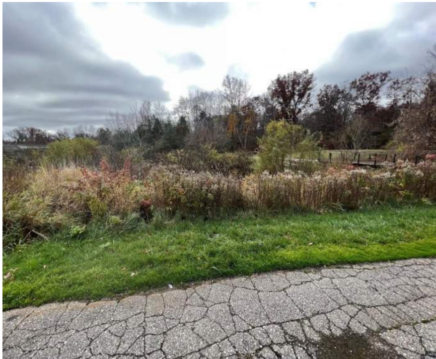
Photo No. 32 – Downstream of Right Embankment – Looking Downstream
