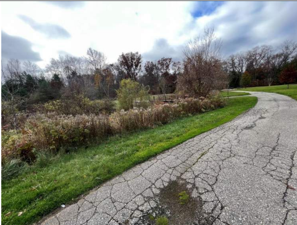
Photo No. 31 – Downstream of Right Embankment – Looking Downstream
