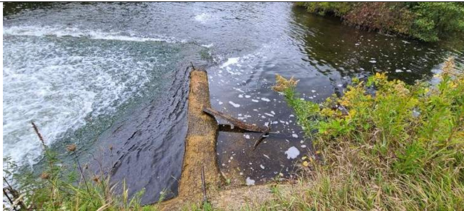
Photo No. 46 – Right Concrete Wall – Downstream of Primary Spillway Looking Downstream
