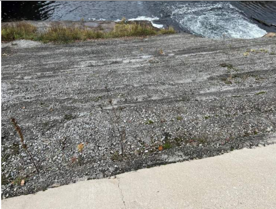
Photo No. 89 – Downstream Left Embankment RCC Slope – Looking Downstream
