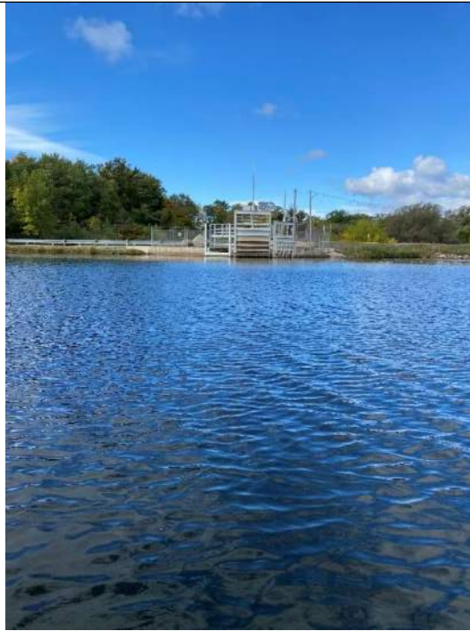
Photo No. 65 – Primary Spillway – Impoundment Looking Downstream
