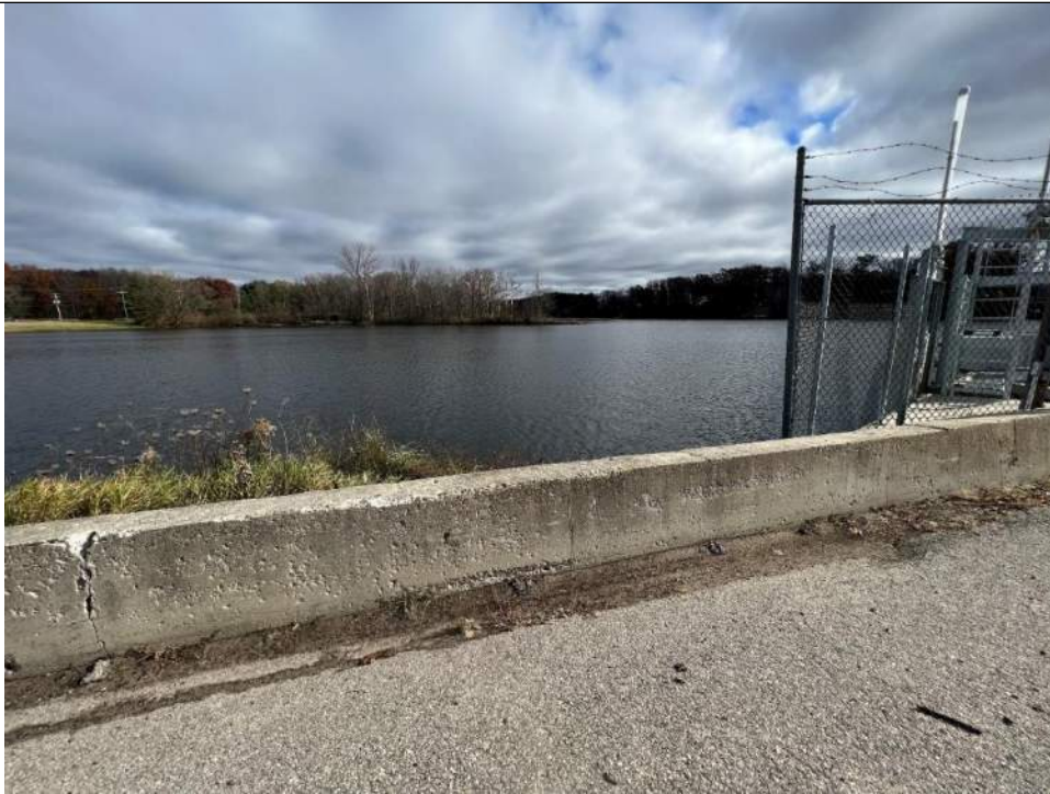
Photo No. 49 – Right Upstream Flood Wall – Looking Upstream
