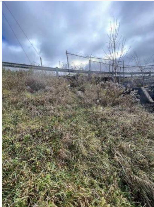
Photo No. 36 – Right Embankment and Right Primary Spillway Wall - Downstream of Road
