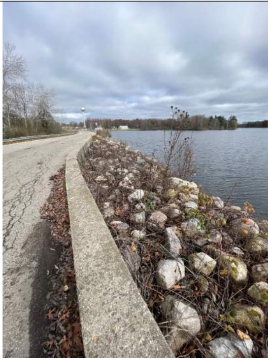
Photo No. 81 – Upstream Left Embankment Flood Wall - Looking Right
