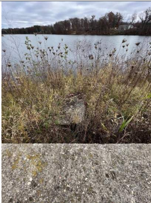
Photo No. 74 – Upstream Left Embankment at Flood Wall Adjacent to Overtop Section – Looking Upstream
