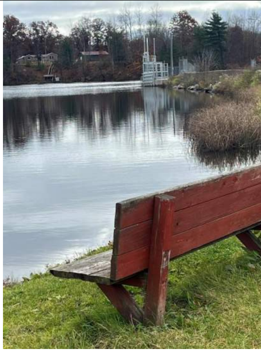
Photo No. 21 – Primary Spillway – Right-Side from Boat Launch
