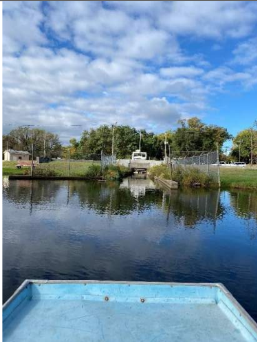
Photo No. 16 – Auxiliary Spillway – Impoundment Looking Downstream
