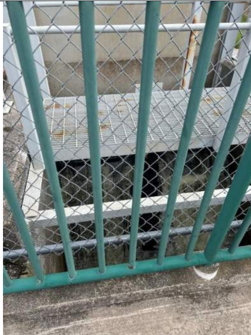
Photo No. 2 – Auxillary Spillway – Operator Walkway Looking Upstream
