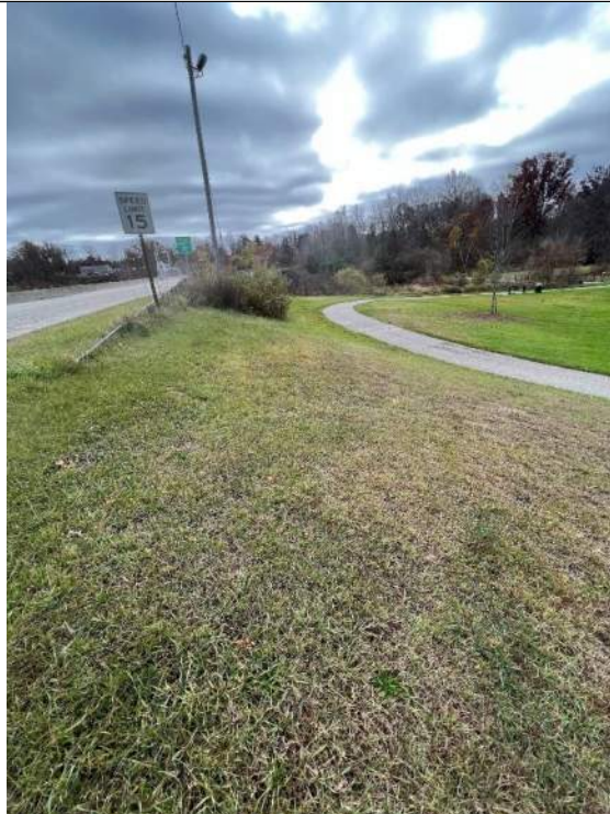
Photo No. 22 – Right Embankment – Downstream Toe Looking Left
