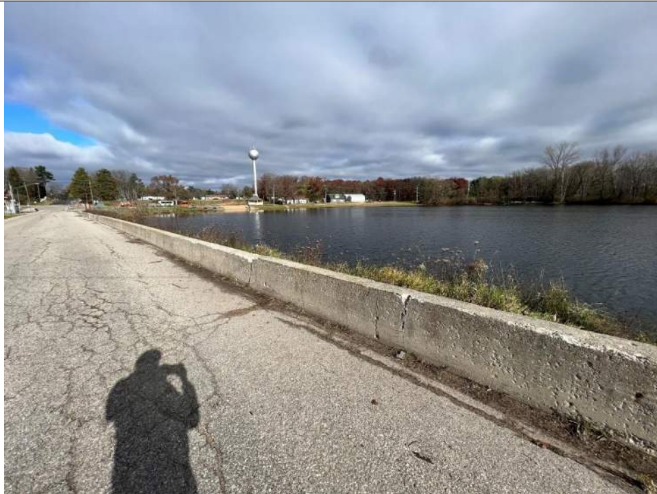
Photo No. 48 – Right Upstream Flood Wall Looking Right
