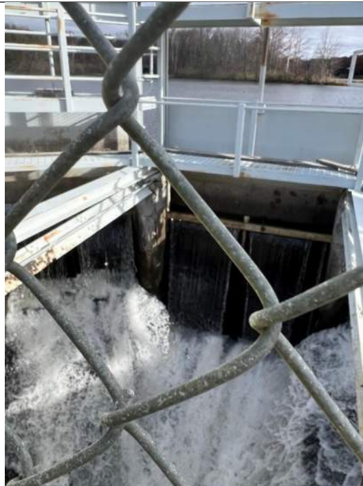
Photo No. 60 – Middle Gate of Primary Spillway – Looking Upstream
