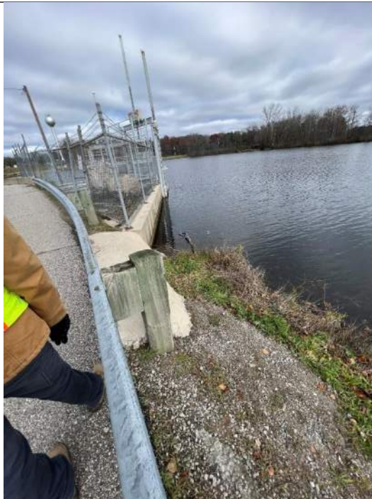
Photo No. 62 – Left Primary Spillway Abutment – Looking Right
