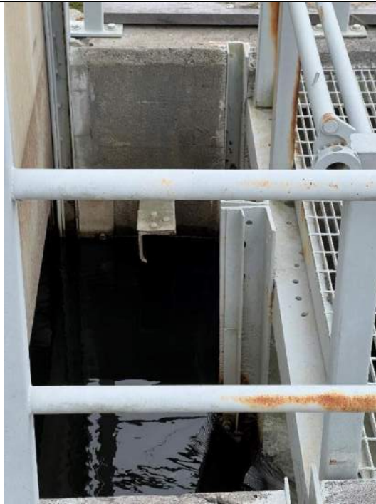
Photo No. 5 – Auxillary Spillway – Gate and Operator Deck
