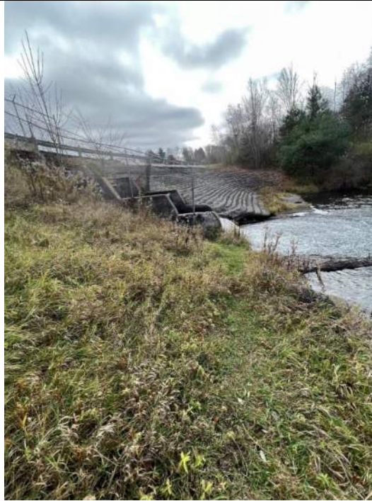
Photo No. 35 – Primary Spillway – Right Wall Downstream of Road
