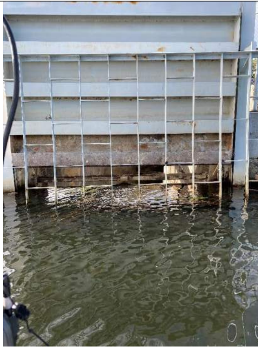
Photo No. 67 – Middle Primary Spillway – Impoundment Looking Downstream
