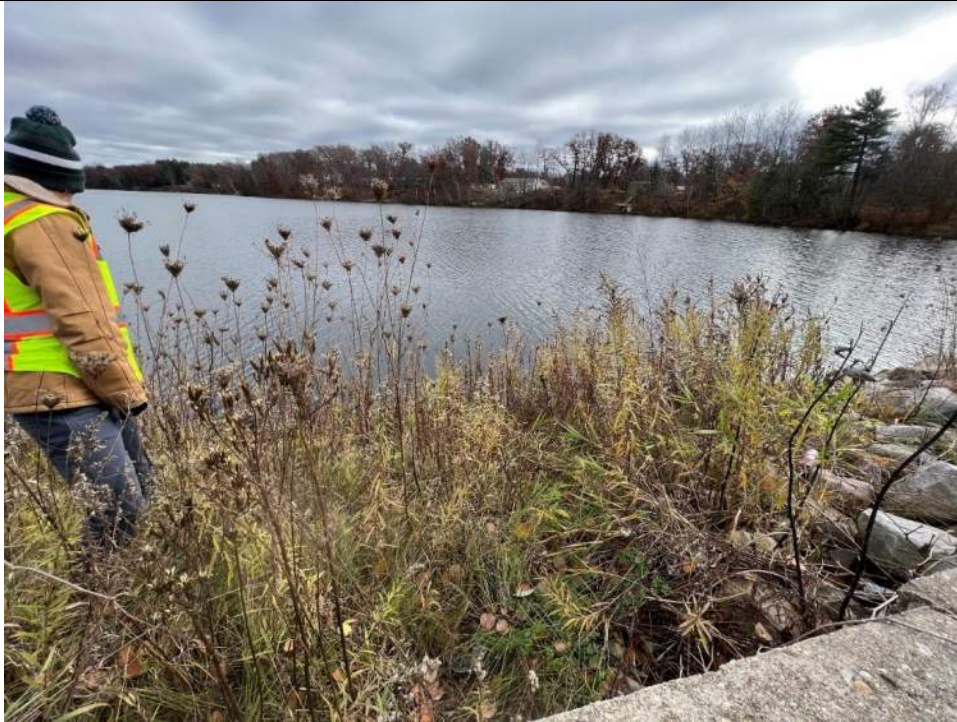
Photo No. 77 – Upstream Left Embankment Flood Wall Transition to Riprap - Looking Upstream
