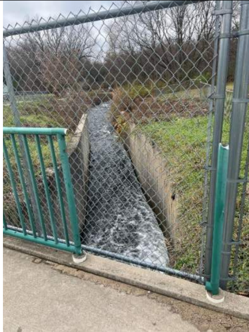
Photo No. 1 – Auxillary Spillway – Downstream of Road Looking Downstream
