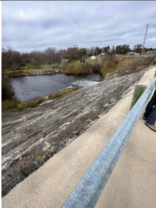
Photo No. 86 – Downstream Left Embankment RCC Slope – Looking Downstream
