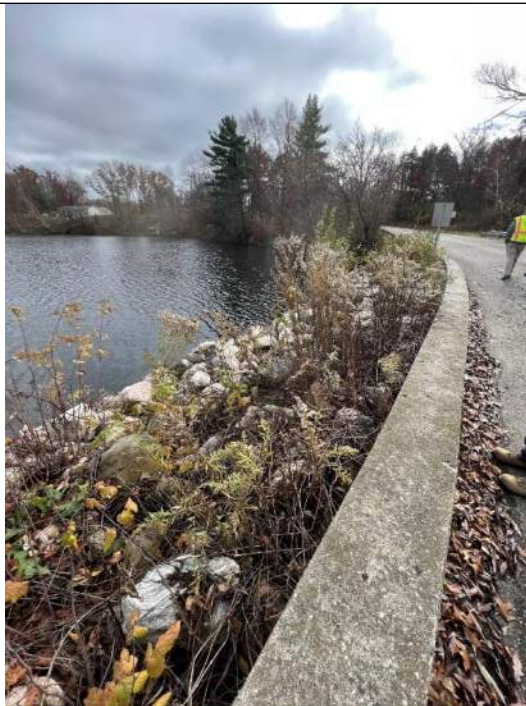
Photo No. 80 – Upstream Left Embankment Flood Wall - Looking Left
