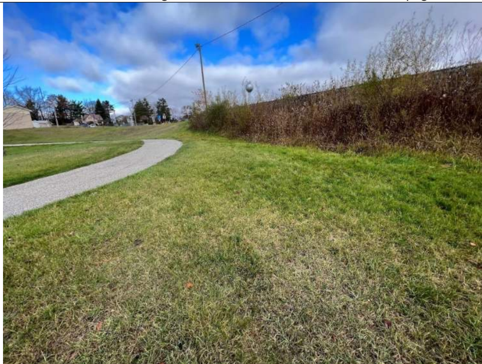
Photo No. 28 – Right Embankment – Downstream Toe Looking Right
