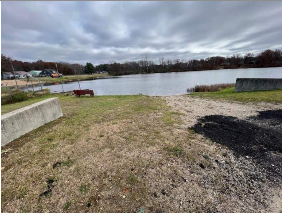
Photo No. 19 – Boat Launch – Looking Upstream
