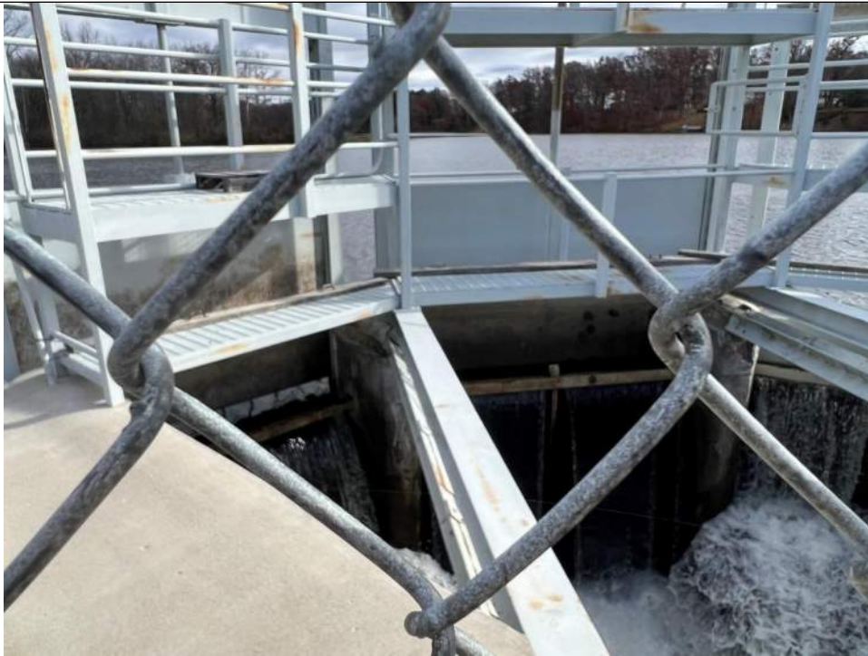
Photo No. 57 – Right Primary Spillway Brace – Looking Upstream
